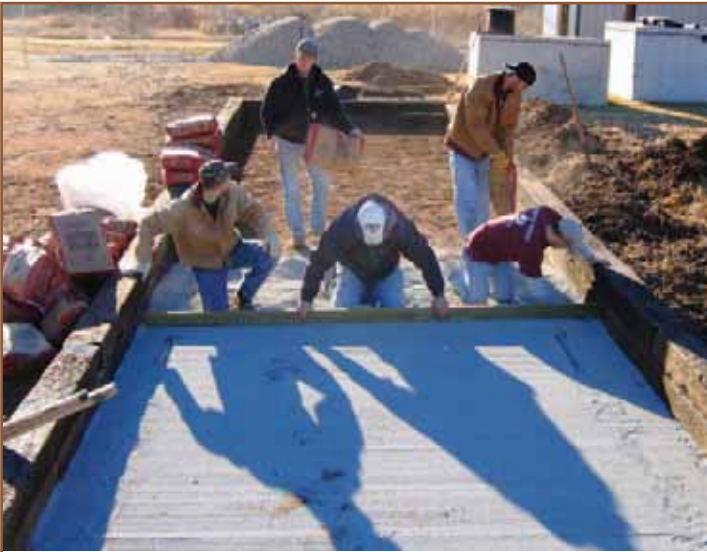
Placing bentonite clay below the wetland liner
