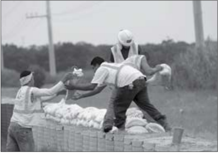
Workers in Port Sulpher, La., stack sandbags on top of retaining wall baskets on Monday preparing for Tropical Storm Isaac.
