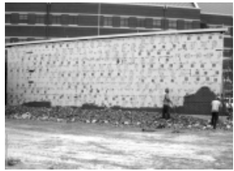
Removing brick from existing building
