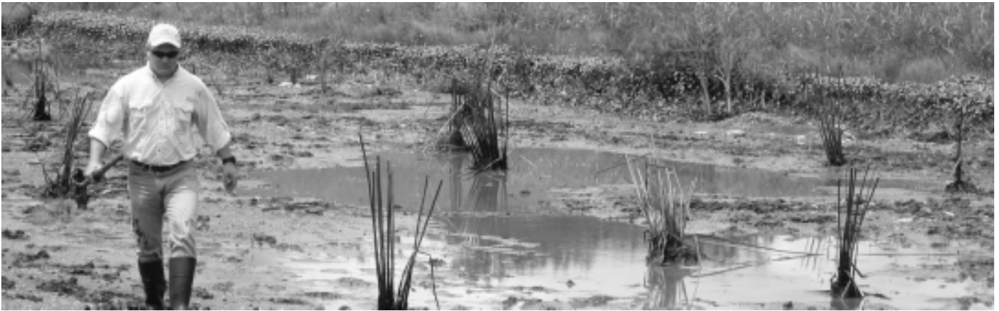
Bruce Byars planting bulrush in the Whitney wastewater treatment
