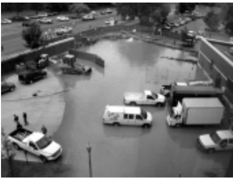
Geo Lake - An unmarked waterline.
