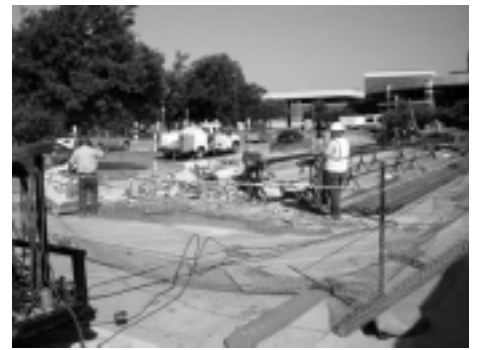
Installing new utilities pipes
