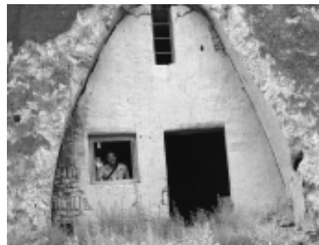
Yardong: You can find these all over the plateau. They are typically found along or below paleosol layers. The enrichment of clay from soil weathering has reduced the permeability and acts as a natural “waterproofing”.
