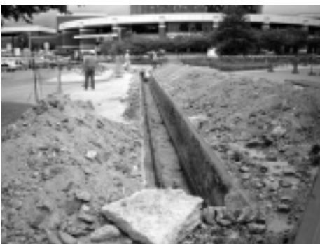
New utilities pipes
