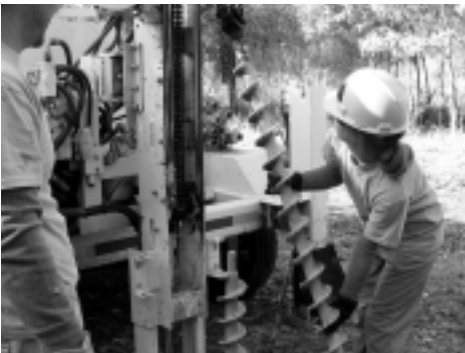
Stephanie Capello adds an auger flight during a piezometer installation at the Waco Wetlands
