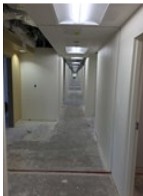
2nd floor side wing corridor with new sheetrocked walls (no more 1-inch tiles!), new lighting, and new window at far end of hallway to provide more ambient light
