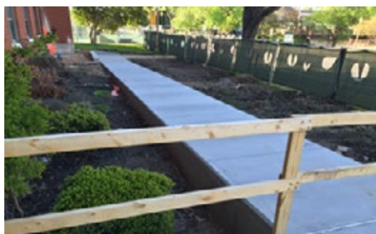
Hardscape going in on exterior of building (new ADA access ramp to front entry for the first time)
