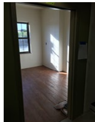
Student rooms taking shape—sheetrocked, painted, new vinyl plank flooring installed
