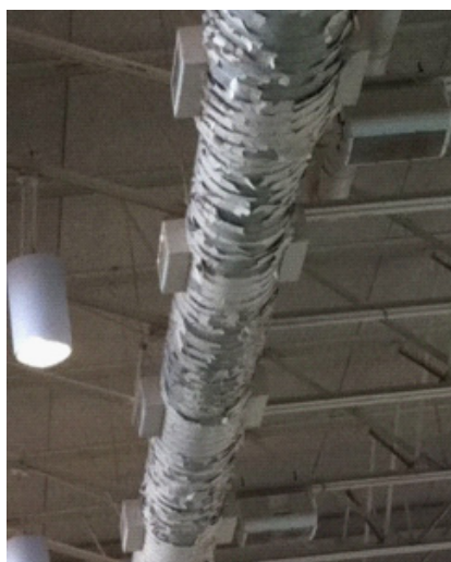
Repainting the duct work (before and after)
