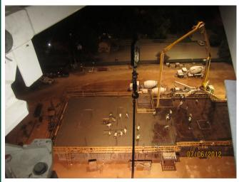
This is a nighttime photo taken from the top of one of the cranes of the South Residence Hall 2nd floor slab pour. Construction teams have to pour the concrete overnight (usually starting at about 1 a.m.) in order to catch the lowest temperatures of the day, since the Texas heat of the day prevents the concrete from "setting up" in a stable fashion if it is poured during the heat of the day.
