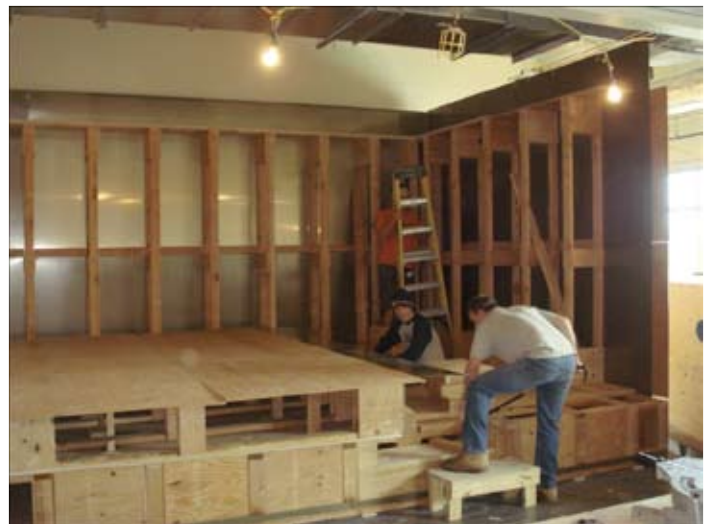
Figure 8. Lifting the third outer shield wall into place.
