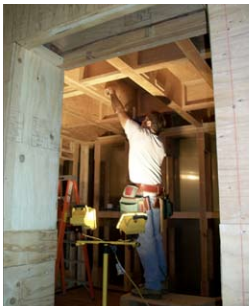
Figure 12. Construction of the inner shield ceiling.
