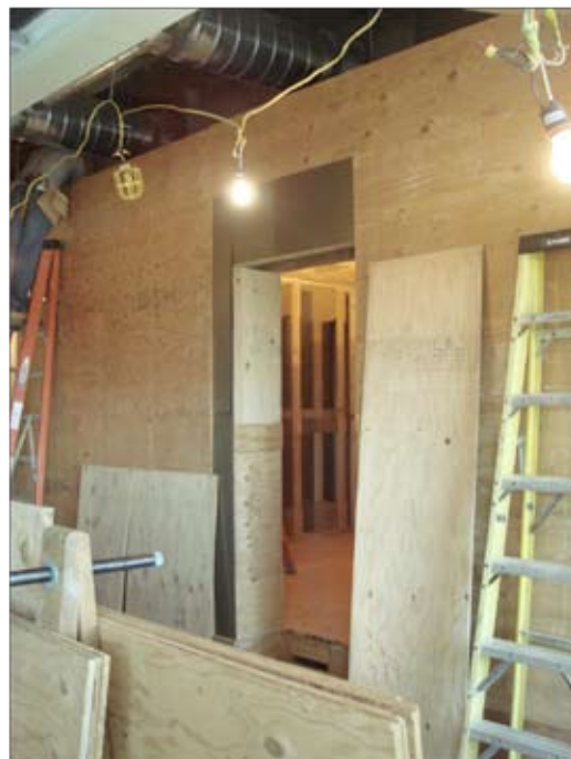
Figure 9. Completion of the outer shield and just prior to demagne- tization of outer shield wall.
