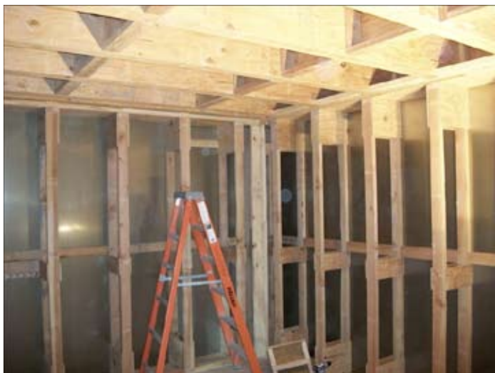
Figure 10. Construction of inner shield walls.
