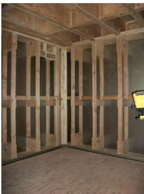
Figure 12. Construction of the inner shield ceiling.
