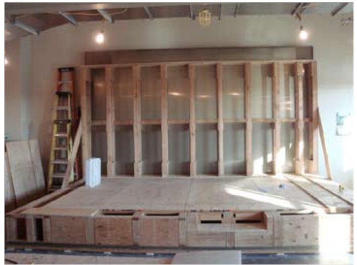
Figure 7. The first outer shield wall and floor in place.
